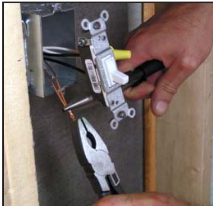
Splicing Ground Wires
