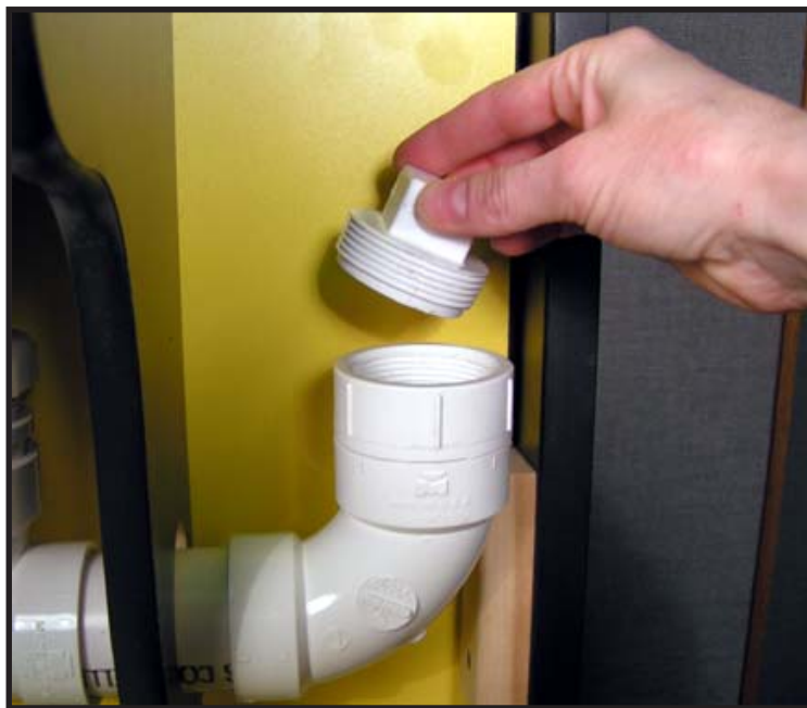
Checking the Clean-Out for Clogs
