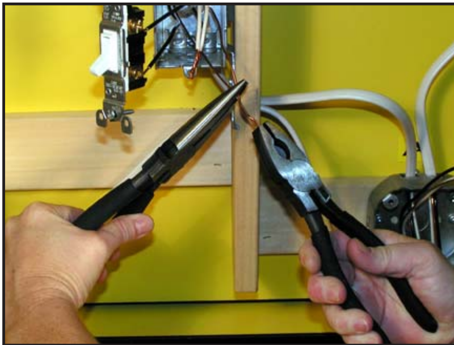
Wiring a Light Switch
